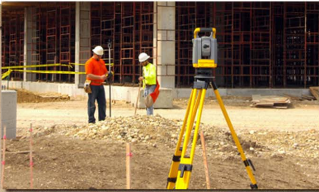
Modern electronic technology such as total stations and GPS can add both productivity and accuracy to construction projects. For extra assurance, it's a good idea to have a trained surveyor check the work of multiple contractors staking on a site. Photo courtesy of R. A. Smith National.
