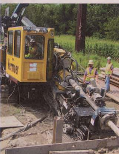
The job includes approximately eight miles of horizontal directional drilling. Left: Vermeer's huge D330x500 was one of the directional drilling machines used.
