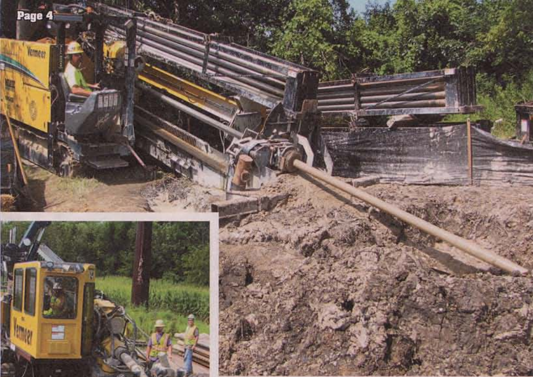
The job includes approximately eight miles of horizontal directional drilling. Left: Vermeer's huge D330x500 was one of the directional drilling machines used.
