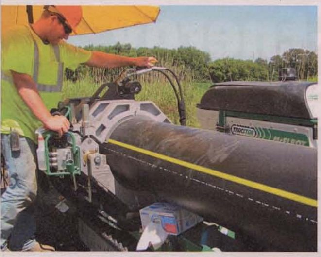
The ends of the pipe are fused together.
